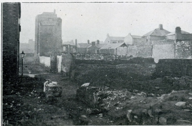
Park Street, showing ruins and waste ground
