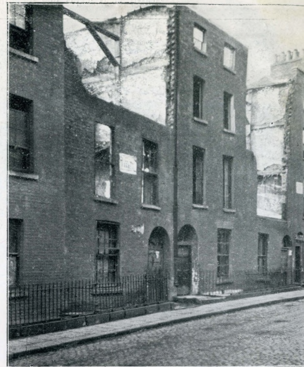
Ruined houses, 68, 69 and 70 Upper Dominick Street.
