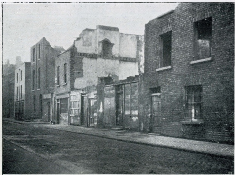
Ruinous houses, 88 to 93 Railway Street.
