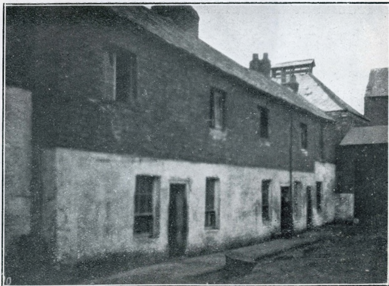
Robinson's Cottages, off Cork Street.
