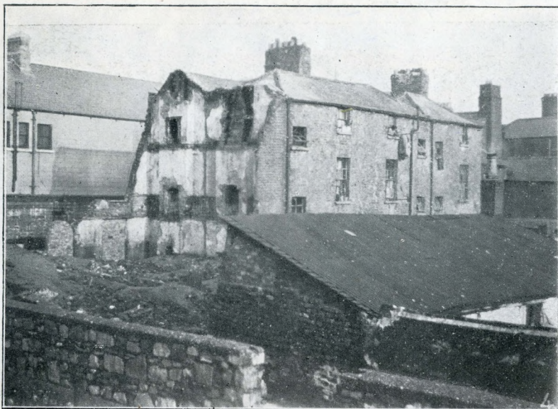
Ruins and dilapidated buildings, Railway Street.
